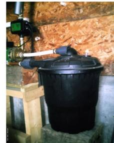
I spent a long time puzzling over the pump aspect. We needed to pump the water up to the header tank in the loft, and we had to make sure it stopped when the header tank was full. I considered using two float switches, one at the top of the header tank for 'off' and one near the bottom for 'on', but the wiring was going to be
