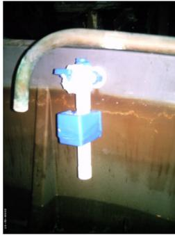
We found a valve that has a float that is constrained to move vertically, and so doesn't 'hunt', and this has been successful, although we've had a couple of occasions when the fact that the pressure has gone down hasn't registered with the pump – and suddenly the hot taps run dry.
