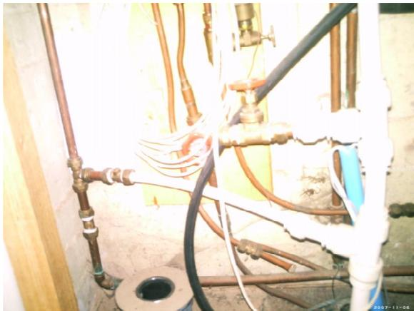
*Rainwater comes in through the white pipe at the bottom right, and goes straight up to the header tank in the loft. Lower white tee-piece leads to stop-cock and copper tee-piece, with mains water coming in through the copper pipe running along the bottom of the photo. Copper pipe going out of the top left leads to the washing machine*
