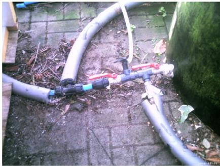
We chose the tank from which we would actually take the water simply because it was closest to the duct that we had laid in years ago, connecting the house to the barn. The water had to be filtered, and we fitted a strainer (small Y-piece seen here on the right), to catch larger bits, and then a garden pond filter.
