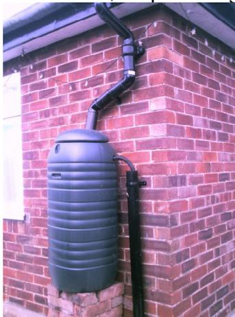
We've extended our catching area, by placing water butts around the bungalow, which are also linked to the main tanks. They don't hold a lot of water; their prime purpose is to catch rainwater from the bungalow and allow it to feed into the other tanks. All of the tanks are arranged so that the tops are at the same level, so that they are all full at the same time. With them all connected, if one was lower than the others, it would overflow, and bring the others down to its level.
