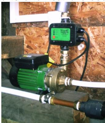
complicated - it meant leading wires from the float switches to the pump, which was going to be in the barn. Then a friend suggested using a shower pump, which automatically stops when the pressure in the pipe builds up. Excellent! But we had to change the ball valve in the header tank, since a normal ball valve tends to 'bounce around' a bit as it fills, which would lead to the pump stopping and starting several times as it neared the top.
